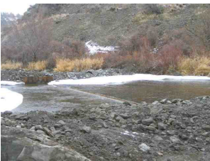
Banks diversion before and after. The banks diversion was a gravel push up dam that reduced water quality due to its installation and constant maintenance throughout the irrigation season.
