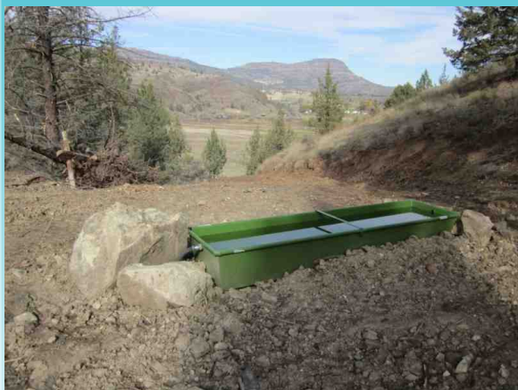
Typical trough installation in conjunction with development of a spring site. This small grant project was funded by Oregon Watershed Enhancement Board.
