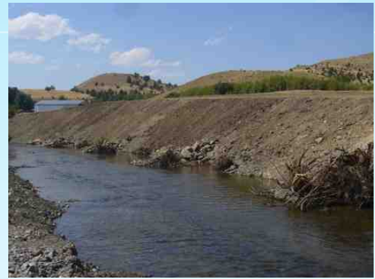
Before and after photos of bank stabilization project on John Day River. Stabilizing the banks reduces bank erosion and sediment in the stream.
