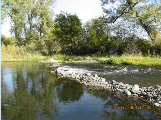
Before and after photos of push-up dam replacement with a permanent lay-down stanchion type diversion structure that eliminates annual stream disturbance.
