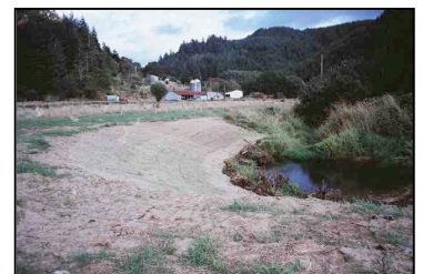
Summer 2010-Excavation and rootwad placement complete
